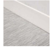
RUBBER BASE | ALLSTATE NO TOE WALL BASE, 2.5" H IN WHITE TYPICAL THROUGHOUT
