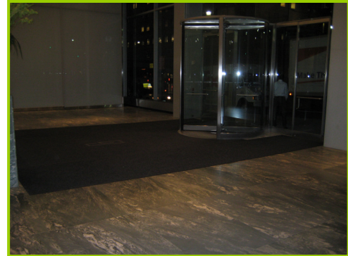
Image 4: Permanent Entryway mats at 100 Park Avenue meet the minimum 10 feet length required for IEQc5.
