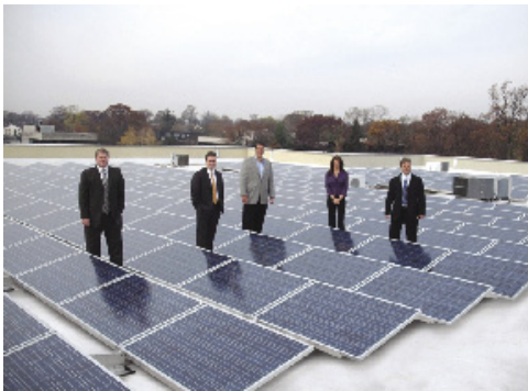
New solar roof located at 500 W. Putnam - Greenwich, CT
